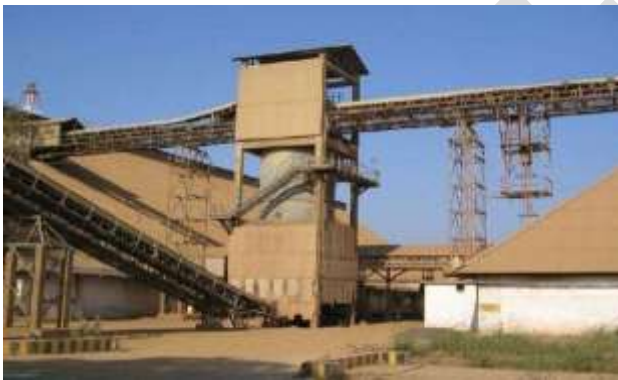
Fig.1.2. Phosphate Rock silo and Conveyance System
